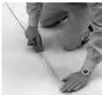
Fig. 3. Butt edges and apply clear, thin packaging tape.
