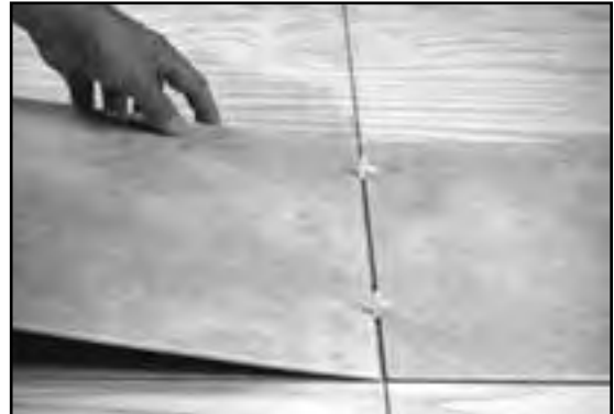
Fig. 13 - Position spacers before setting the tile.
