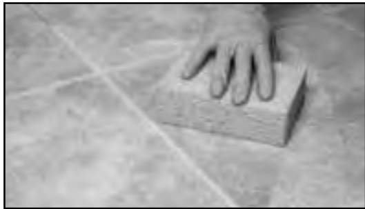
Fig. 24 - Wipe diagonally across the joint to remove excess water.
