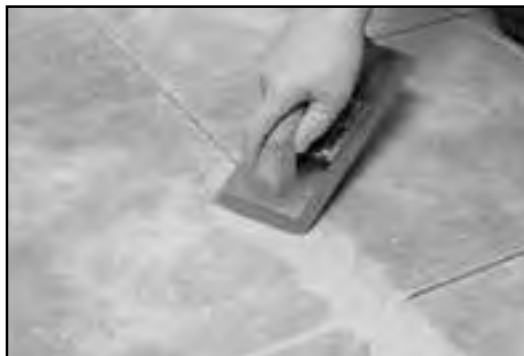
Fig. 21 - Pack the grout into the joints.
