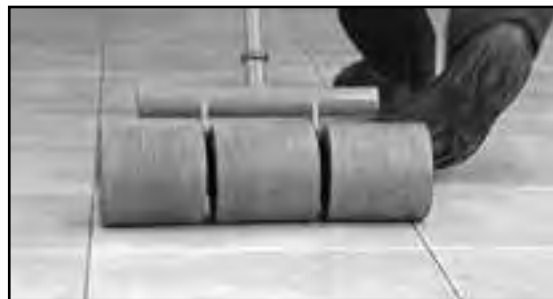
Fig. 16 - Roll the floor within one hour after setting tiles.
