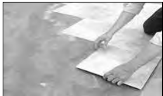
Fig. 15 - Install ungrouted floors following a stair-step pattern.
