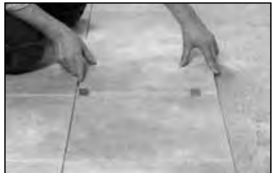
Fig. 14 - Set tile in straight rows.
