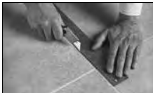
Fig. 25 - Cut along the center of the grout line after heating it.
