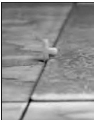
Fig. 12 - Use spacers with one leg removed.
