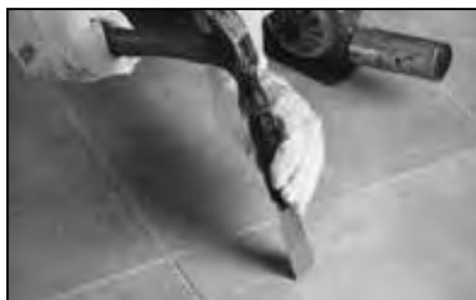
Fig. 26 - Drive a putty knife into the heated area and pry upward.
