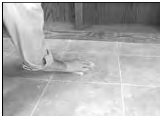
Fig. 23 - Use a 3M white, nylon pad to loosen grout residue.
