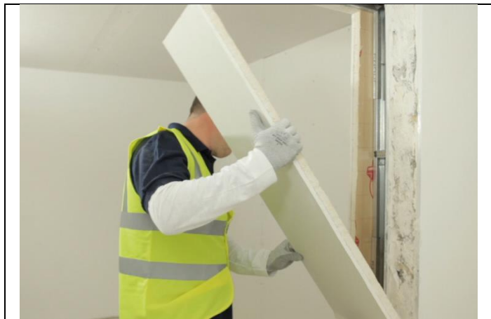
Figure 4 Window reveal installation
