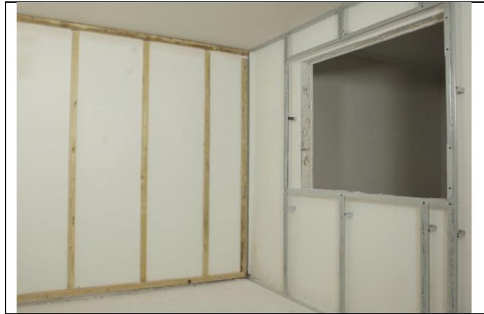
Figure 4 Window reveal installation
