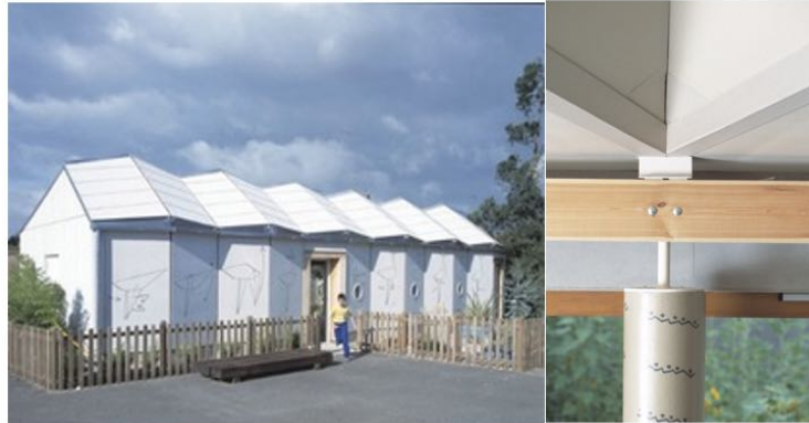
Fig. 6 – Cardboard building for Westborough Primary School and Kindergarten in Westcliff on Sea (UK) (source http://www.engagingplaces.org.uk/teaching%20resources/art67590 accessed 17.03.2020).
