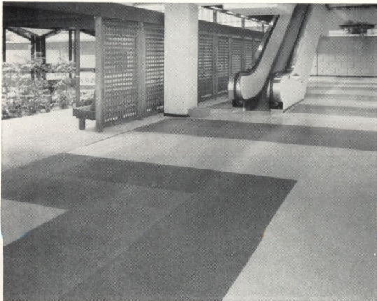
Custom floor designs can be achieved without greatly increasing the cost. Right angles, straight lines, and minimal waste made this striking custom floor cost very little extra.
