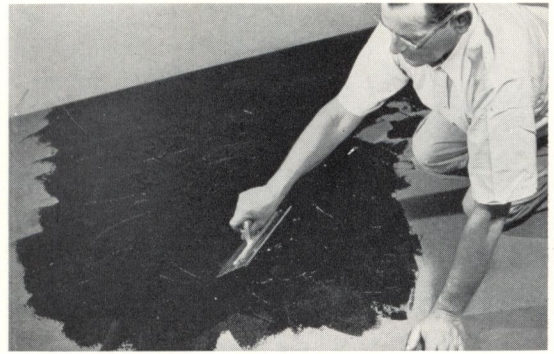
Latex-type underlayments may be troweled to a thin "featheredge" in leveling worn or damaged areas of concrete subfloors. This often eliminates the need for grinding or a complete new concrete topping.
