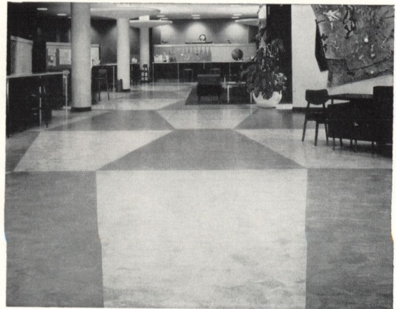
More elaborate custom styling as in the floor above costs more than that on the left due to increased cutting and fitting. Curves and irregular shapes would cost even more.
