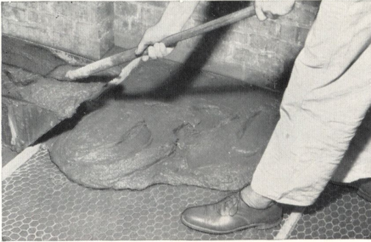
Over wood subfloors, galvanized chicken wire or expanded metal lath should be nailed to the floor to reinforce asphaltic-type underlayments. The wire mesh allows the wood floor to expand and contract without damaging the floor fill.
