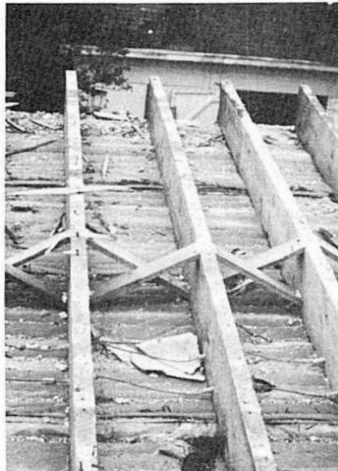
Figure 9. Double ply Cabot's Quilt between floors
