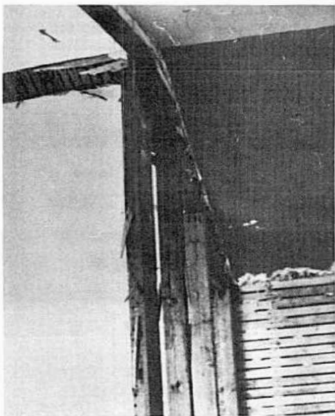
Figure 12. Continuous top plates
