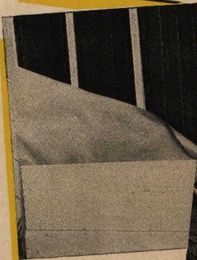
Install vapor proof paper to face of framing members on warm side of wall before applying lath and plaster.
