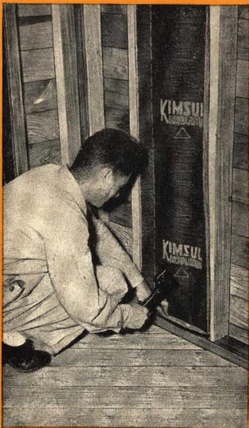
Step 3 —Expand blanket until stitching is taut and nail or staple through strip at bottom.
