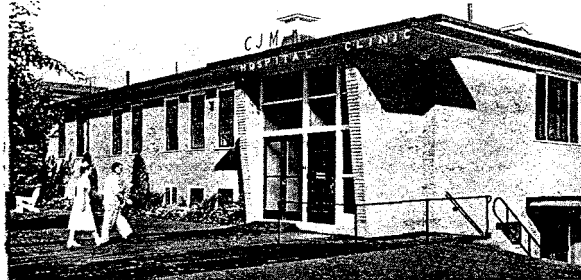
The company-operated hospital and clinic
