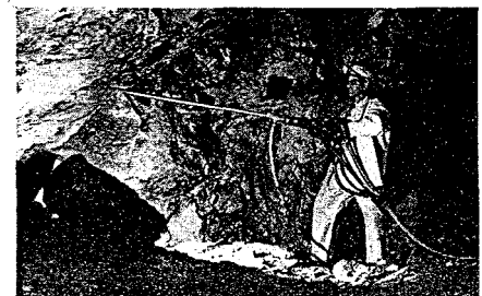
Drilling preparatory to block caving
