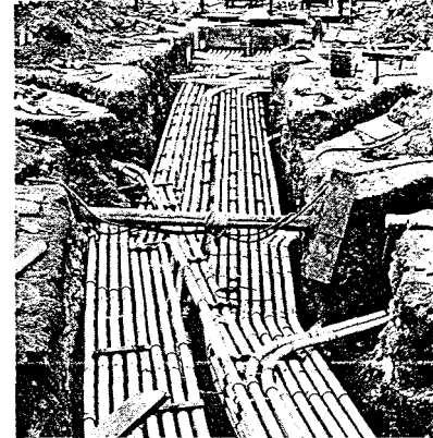
As modern water and sewer mains
