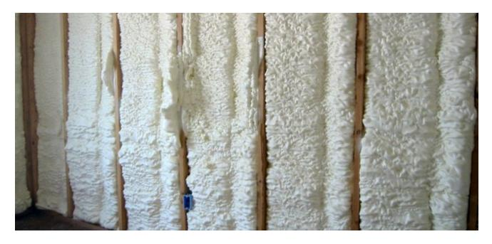
Icynene plastic insulation blown into the walls of a home near Denver. Icynene fills cracks and crevices and adheres to the framing.
