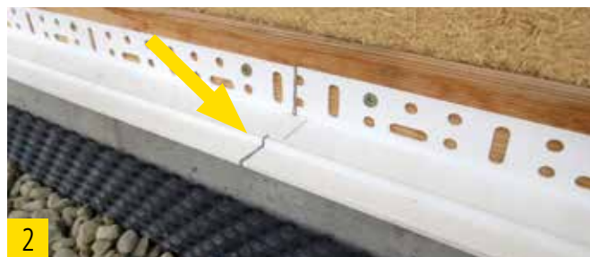
Installation of butt joint connectors at all longitudinal ends.
