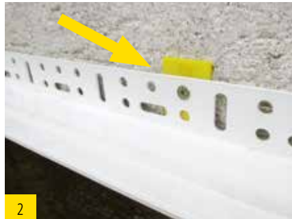
Distance adjustment at the base rail.
