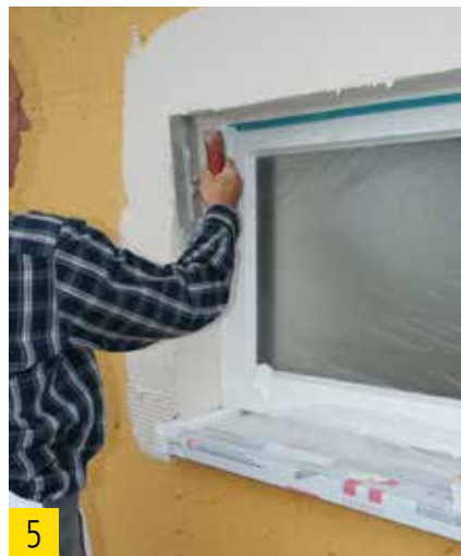
Embedding of the architrave bead with telescope function.
