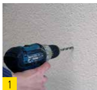
1 Pre-drilling of the rendered wood fiber insulation board by means of an 8 mm wood drill.
