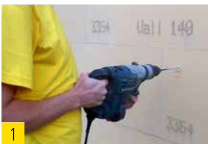
Pre-drilling by means of an impact drill.
