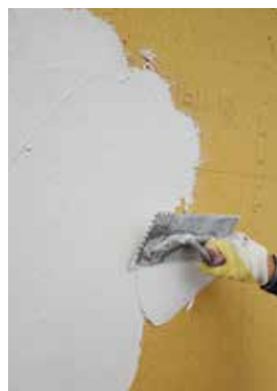
Application of adhesive and reinforcing mortar (UP).
