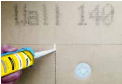
Closing the installation joints by means of FDM WALL.
