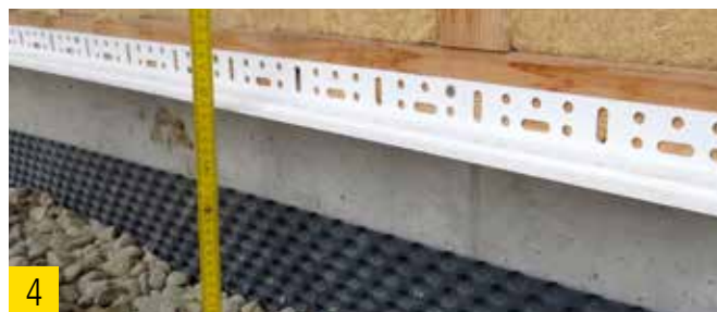
Splash water zone of \geq 30 cm without any additional measures.
