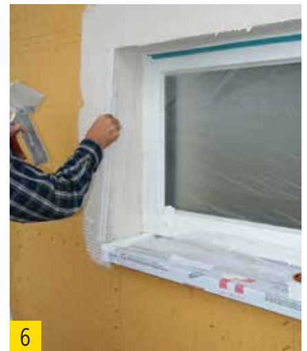
Application of corner bead with fiber mesh.
