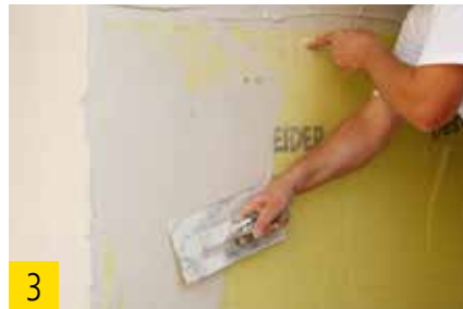
3 Wet embedding of the best wood fiber reinforcement fabric.
