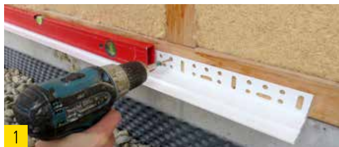
Base rail must be aligned and fastened horizontally.
