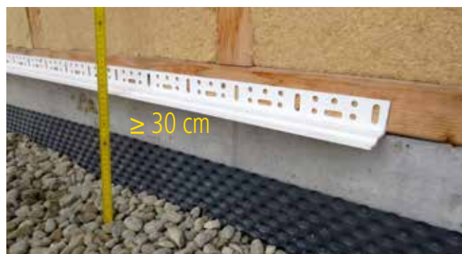
Splash water zone of \geq 30 cm without any additional measures.
