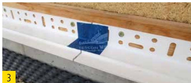
Bonding of the joint by means of a fabric tape.
