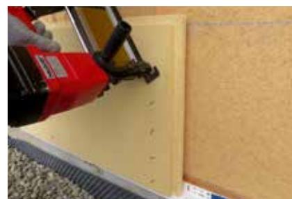
Fastening by means of broad back staples.
