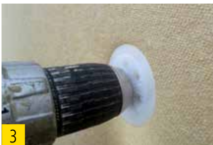
The anchor has to be flush-mounted to board.
