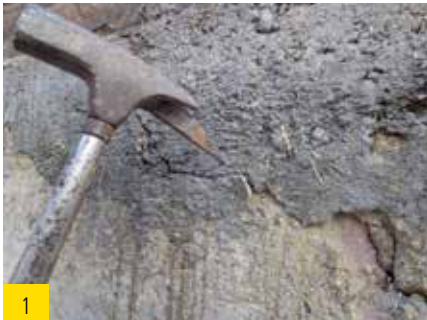
1 Remove all loose plaster.
