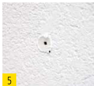
5 Remove any excess FDM WALL between plaster and spiral anchor.
