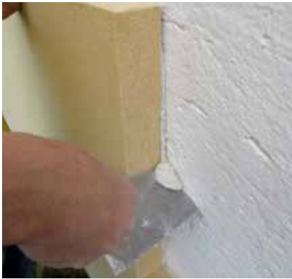
Remove any emerging adhesive.
