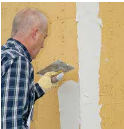
Application of adhesive and reinforcing mortar (UP).
