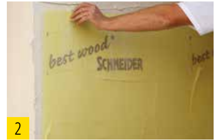
2 Application of best wood fiber reinforcement fabric.
