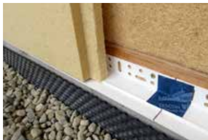
Cut off the groove side.
