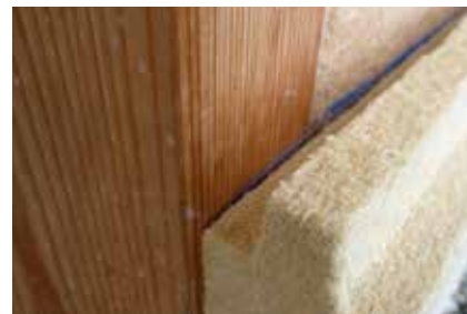
Horizontal alignment of the first row of panels by means of a marking chord.
