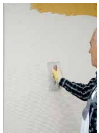
Application of the coating by means of a toothed spatula.
