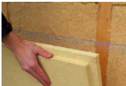
Horizontal alignment of the first row of panels by means of a marking chord.
