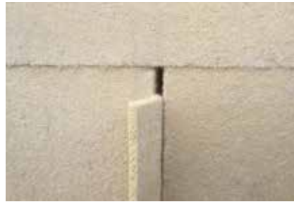
Closing the installation joints by means of strips from WALL 140/180.
