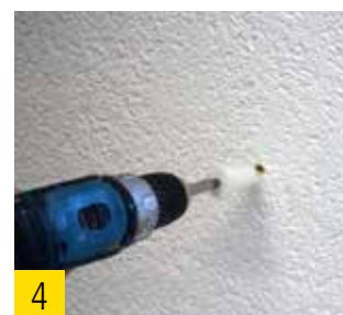
4 Flush insertion of the spiral anchor by means of a TORX T40 into the rendered wood fiber insulation board.
