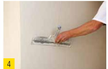
4 Embedding of the best wood fiber reinforcement fabric.
