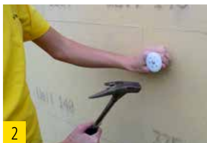
Application of the screw-in anchor.
