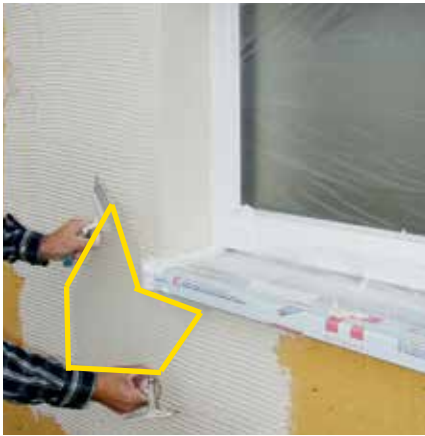
Embedding of reinforcing arrow.
