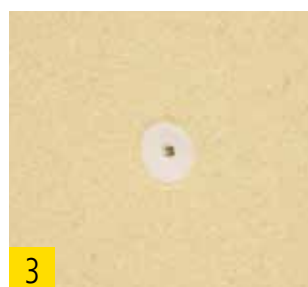
3 Flush-mounting of the spiral anchor.
