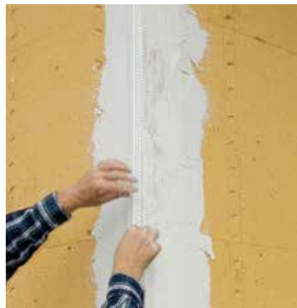
Application of corner bead with fiber mesh.
