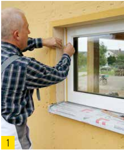
Adhesion of the architrave bead with telescope function.
