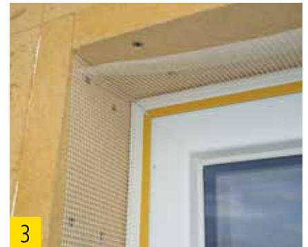
Architrave bead mitered in the edge.
