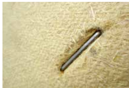
Broad back staples have to be countersunk approx. 1 mm into the best wood WALL 180.
