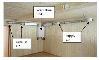
Figure 1: built in mechanical ventilation system in the wooden module
