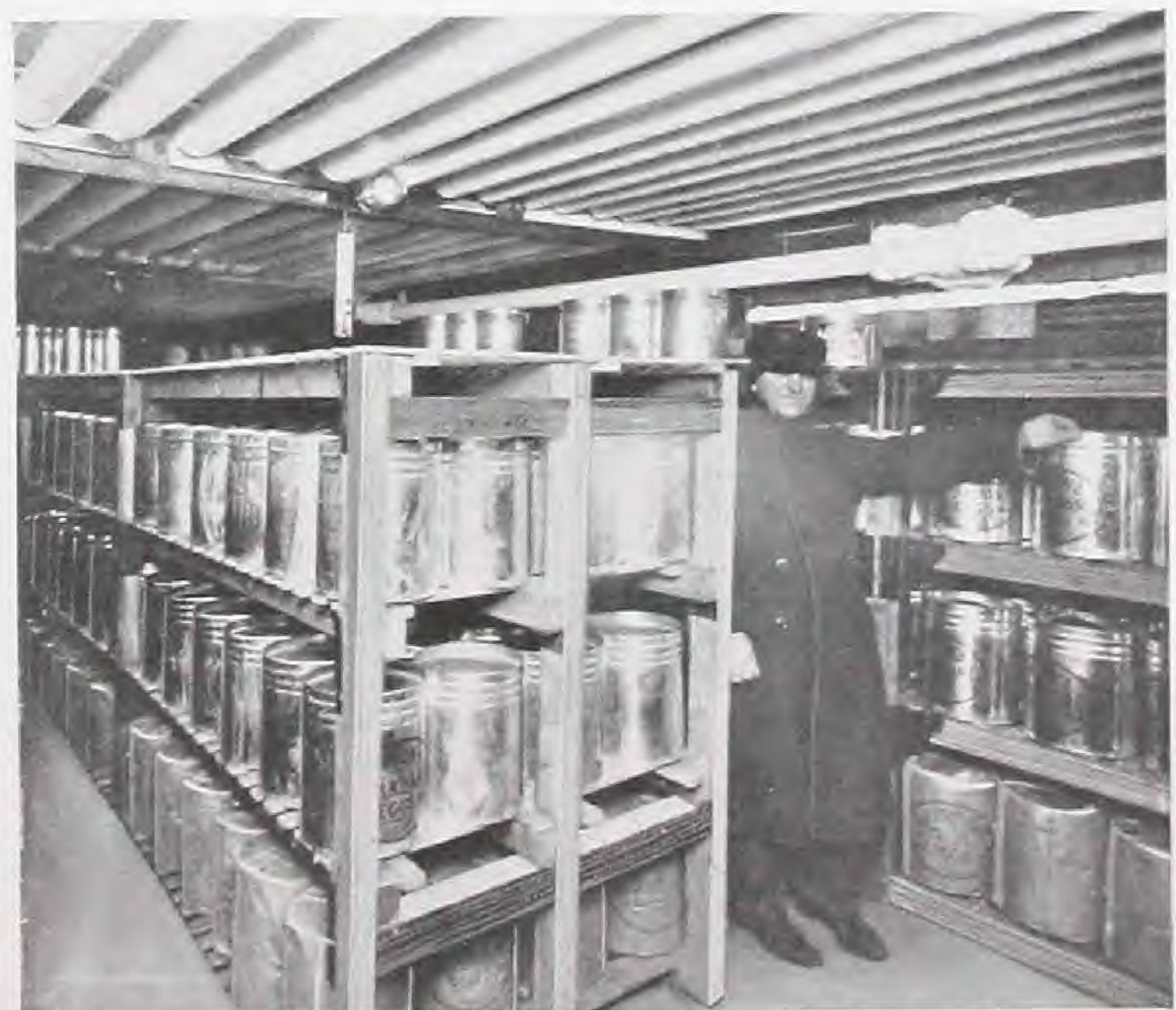
Storage Room in George J. Cooke Co.'s Cold Stores Insulated with Cabot's Quilt. Thermometer shows temperature of -4°
