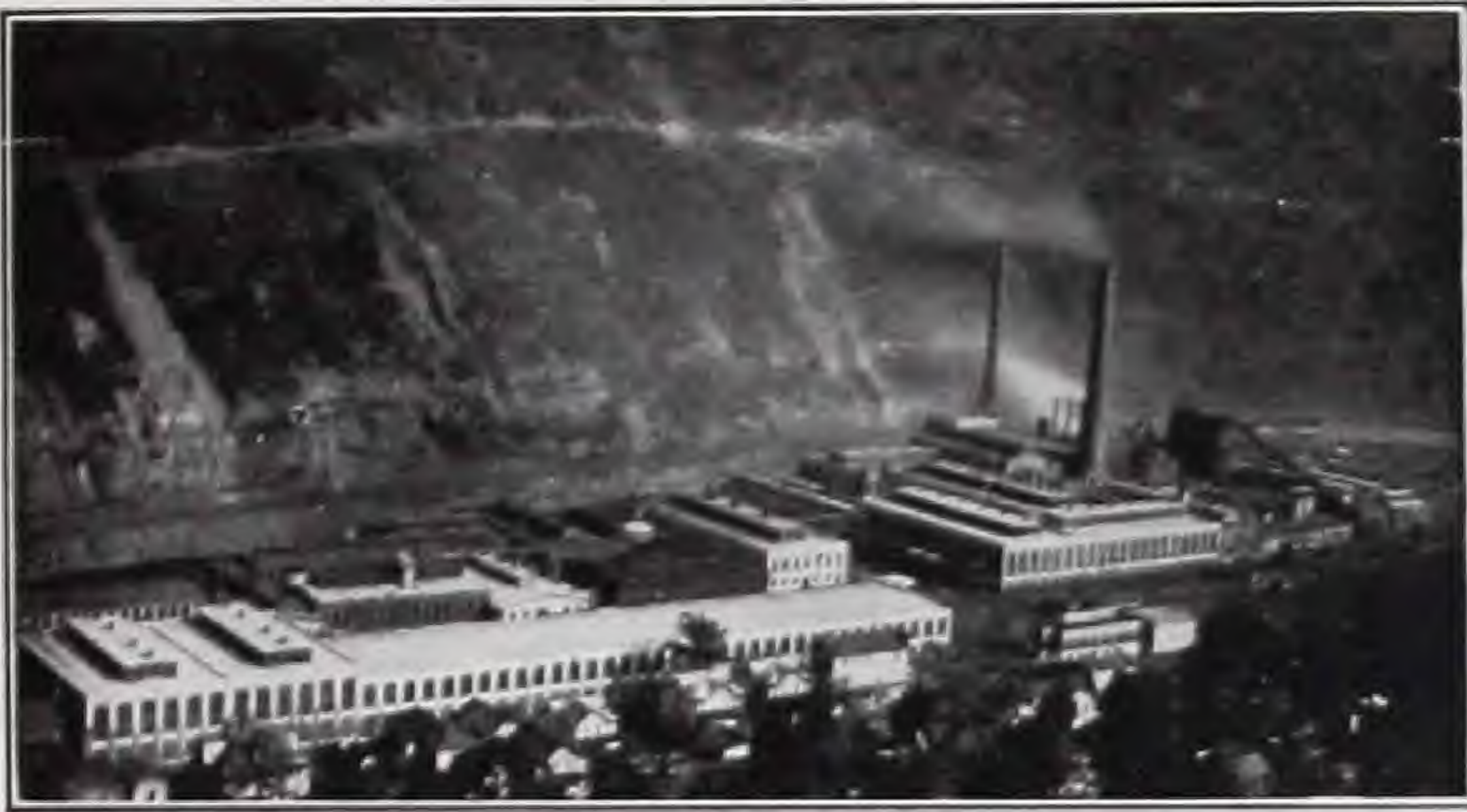
West Virginia Pulp and Paper Co.'s Plant F. G. Ten Broeck, Engineer, N. Y.
