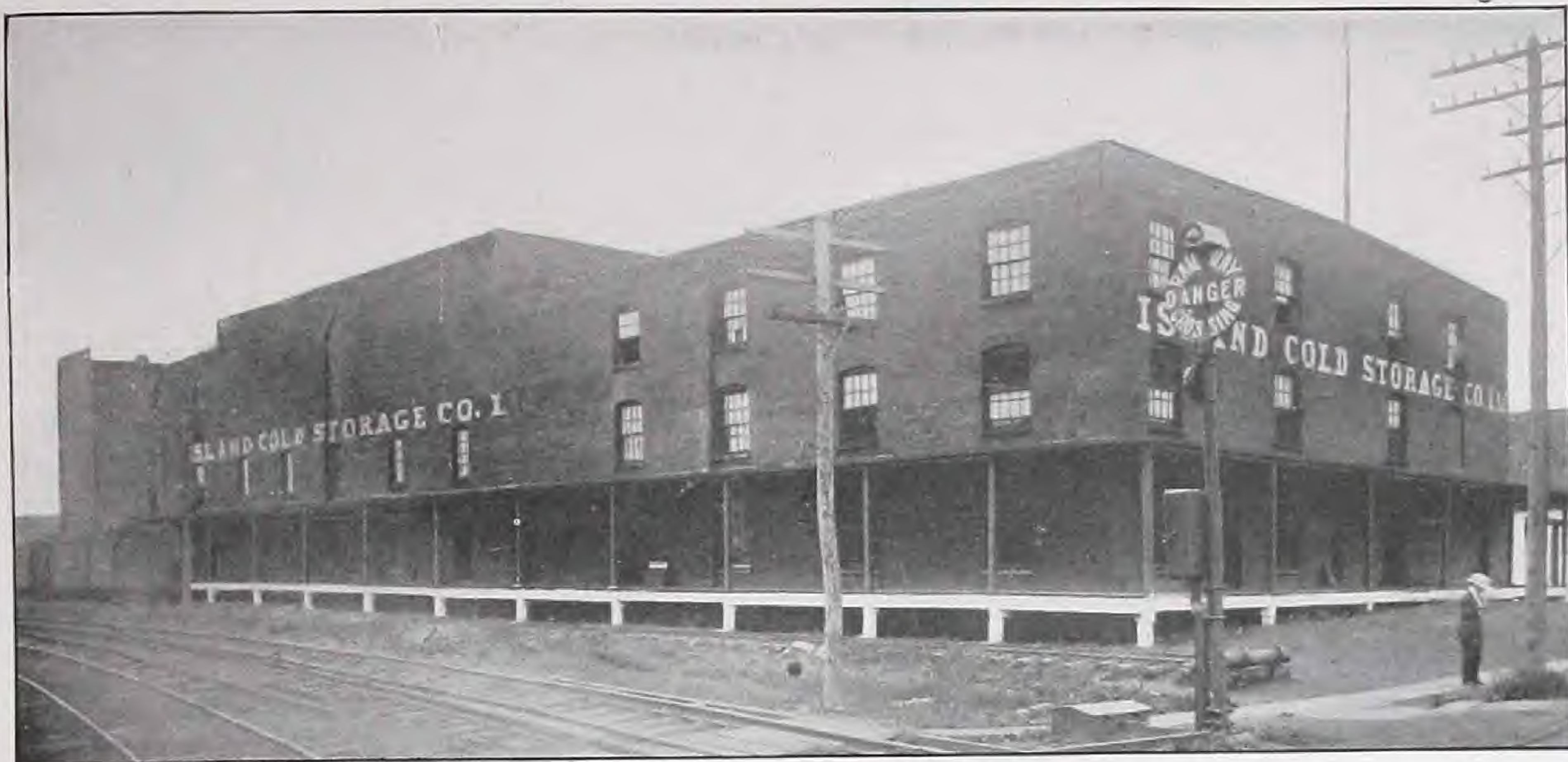
Island Cold Storage Co., Charlottetown, P. E. I. Insulated with Cabot's Quilt to replace cork insulation that had rotted
