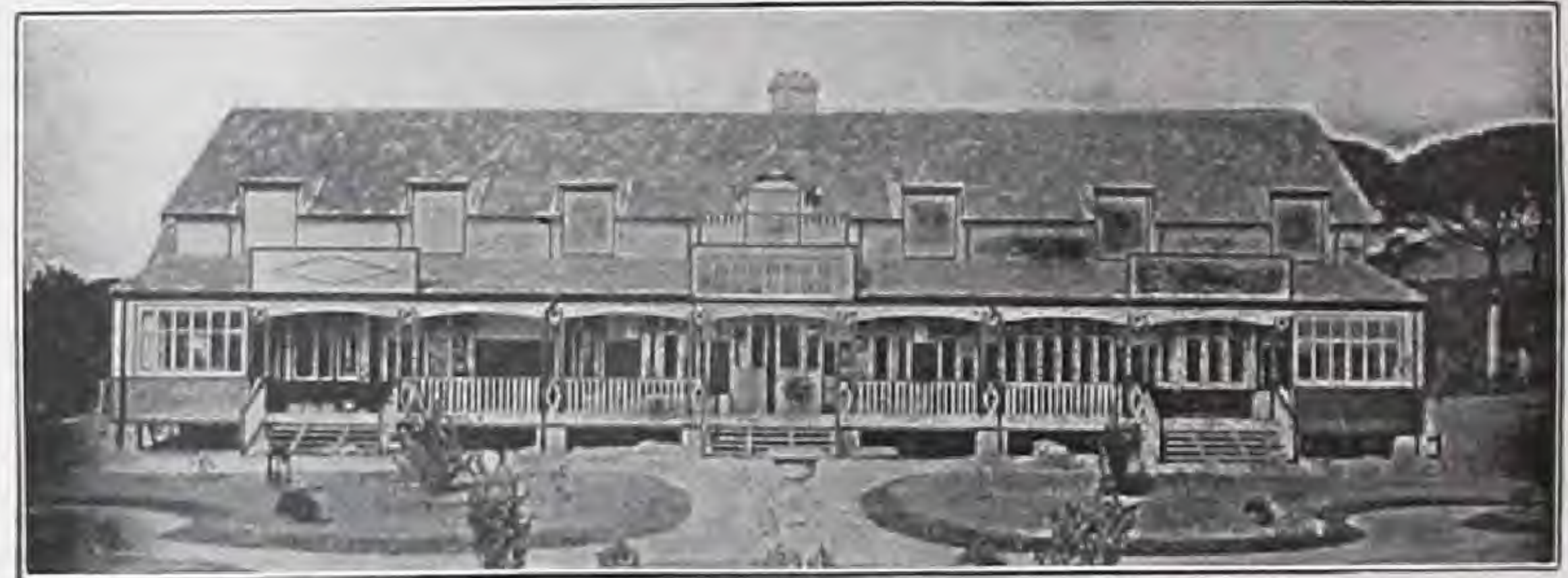
Portable Bungalow Club-house in France Insulated with Quilt
