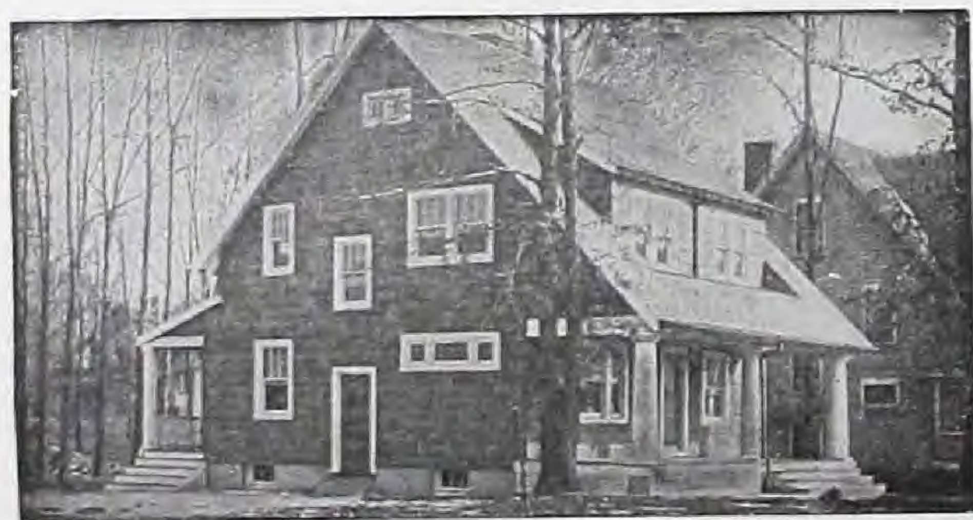
Residence of Walter M. Collins, Builder, Bayside, L. I.
