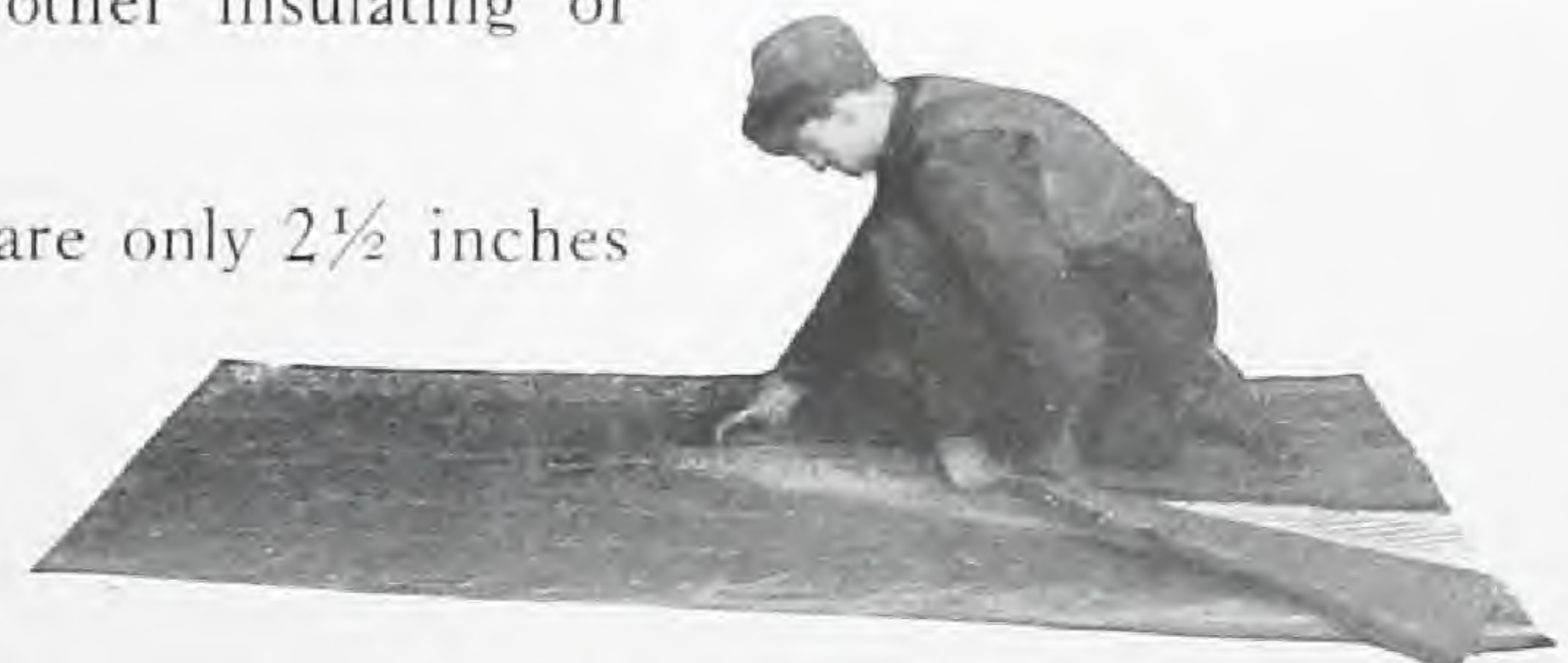
Splitting into Strips with Shears. A Knife Can Also Be Used
