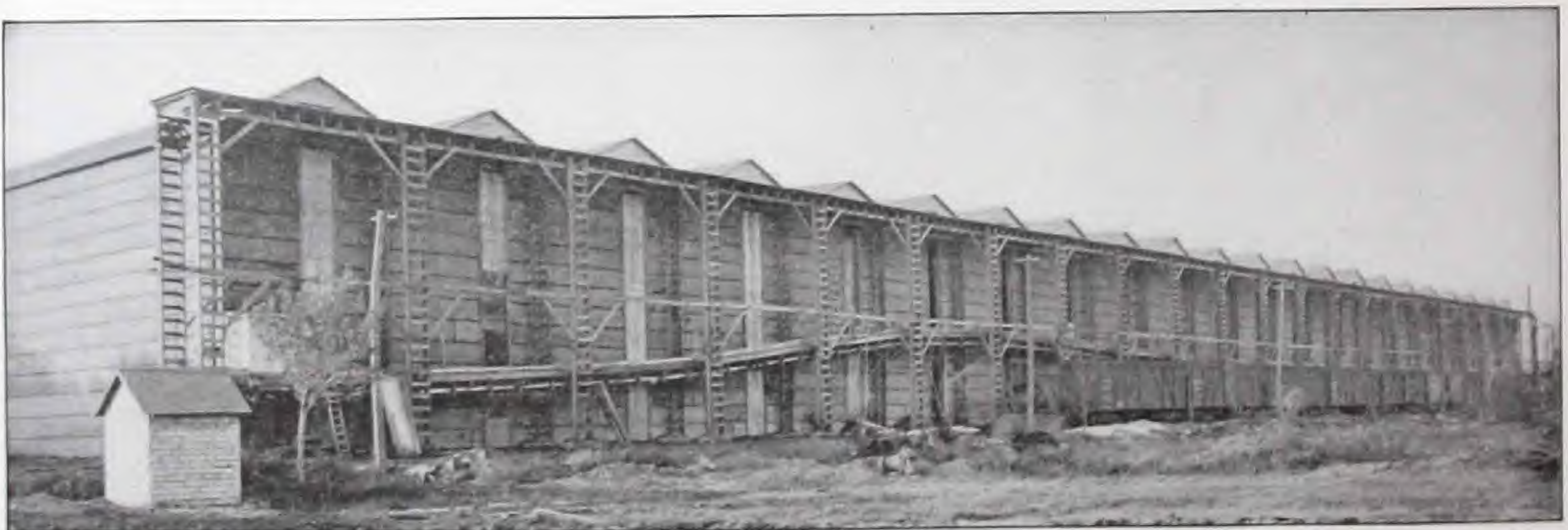
Storage House of The Canadian Ice Co., Limited, Hudson, Quebec
