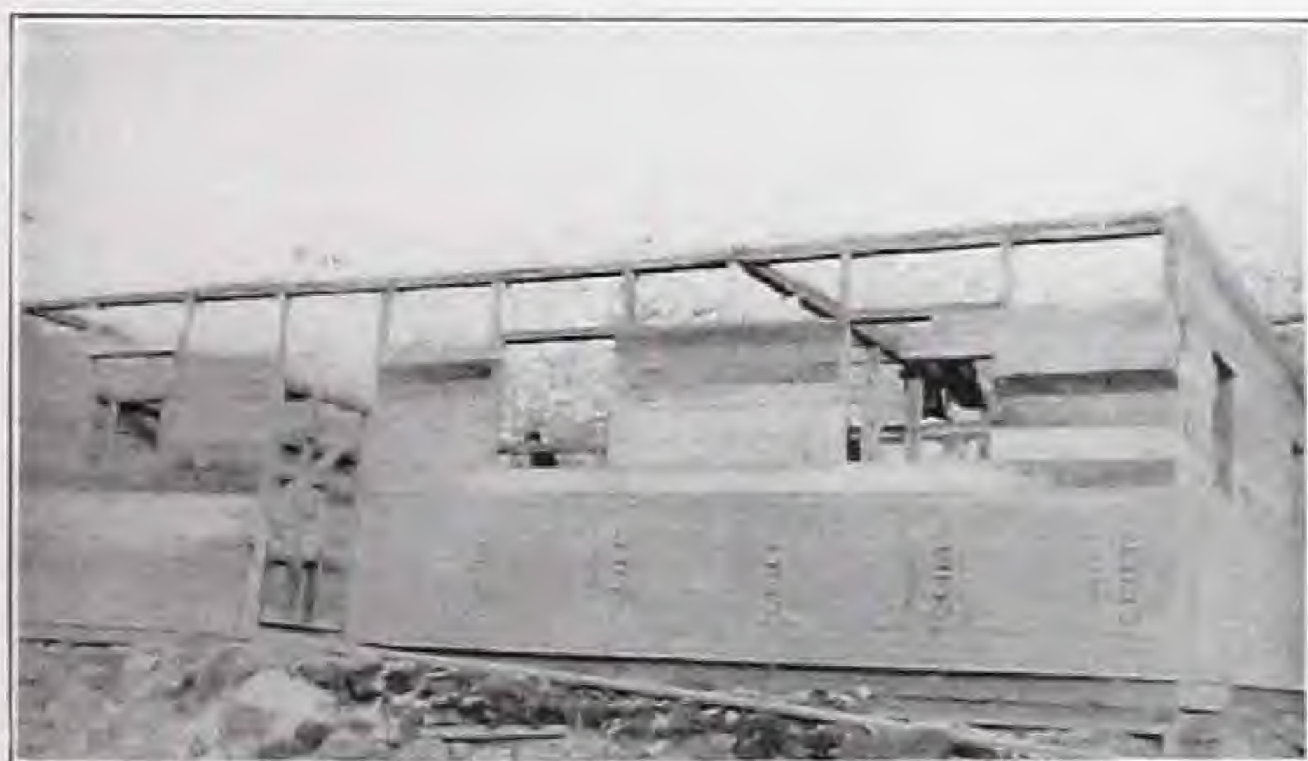
During Building, showing how Cabot's Quilt was applied to Walls
