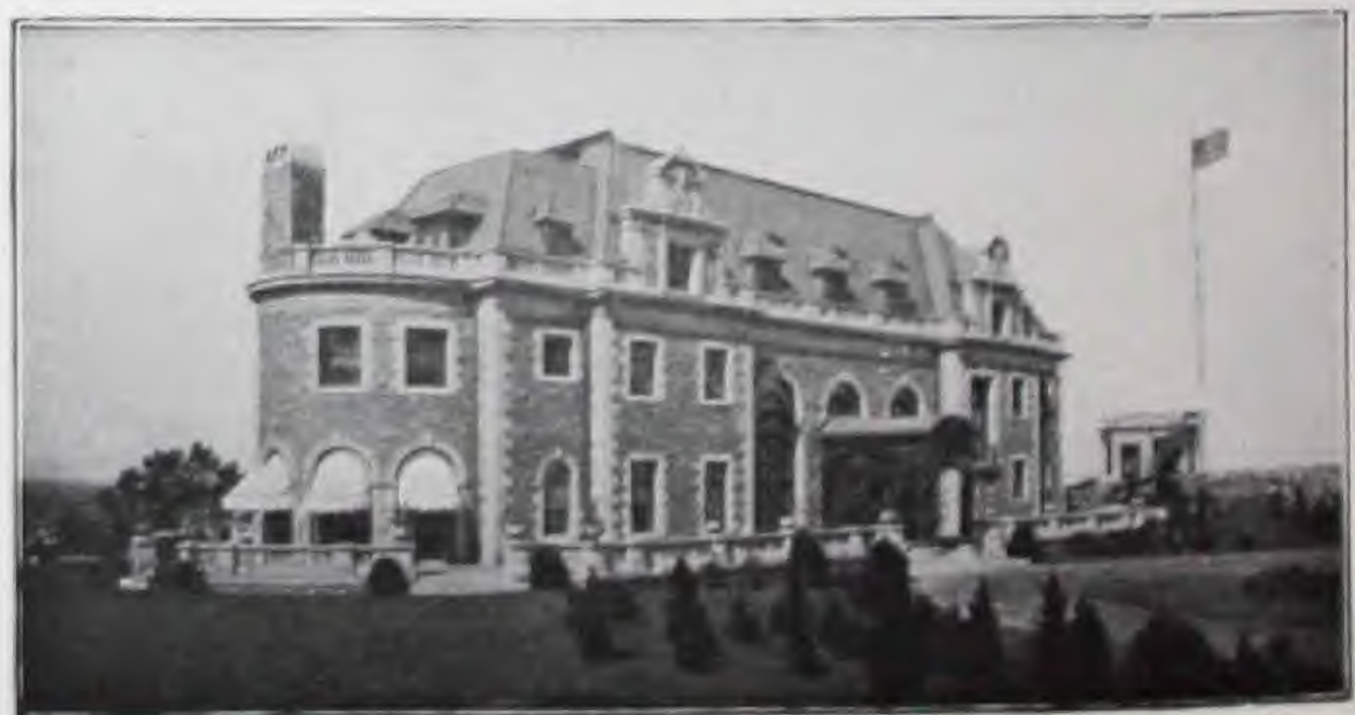
Residence of Arthur Curtis James, Newport, R. I. Howells & Stokes, Architects, New York
