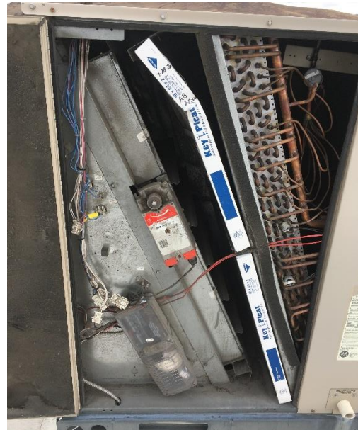
Figure 6. Picture of filter not seated correctly.
