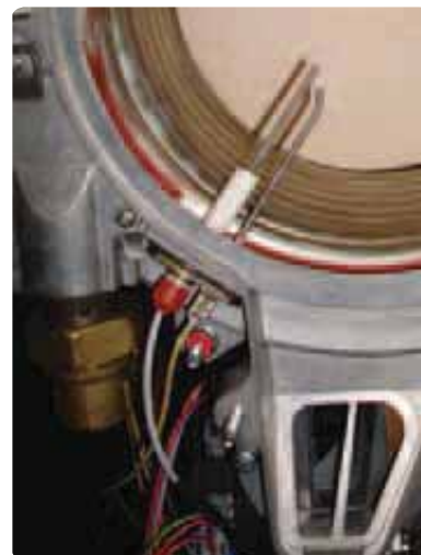
Figure 132 Inspecting ignition electrode
