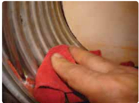
Figure 143 Cleaning the heat exchanger
