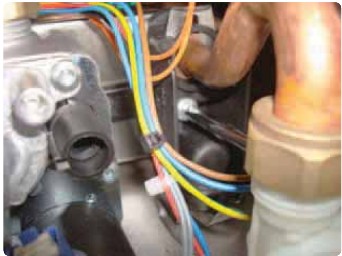
Figure 149 Removal of flat plate heat exchanger (screw on right side)
