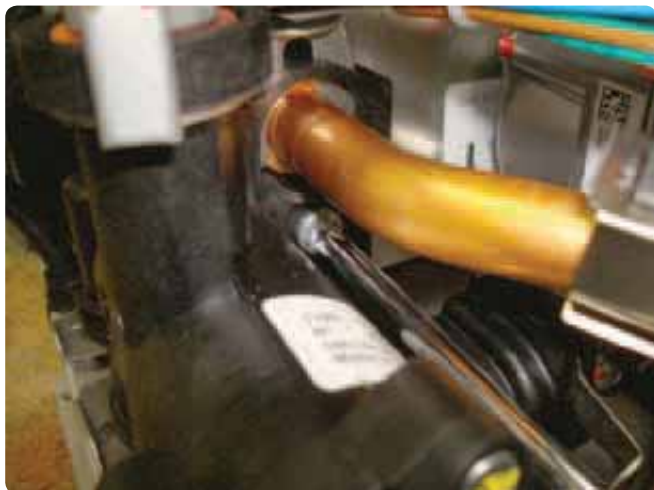
Figure 148 Removal of flat plate heat exchanger (screw on left side)
