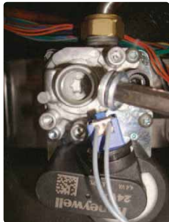
Figure 99 T-40 cap removed for adjustment
