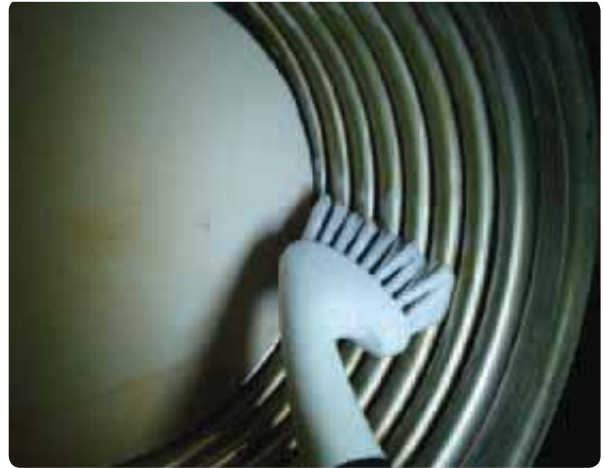
Figure 142 Cleaning the heat exchanger
