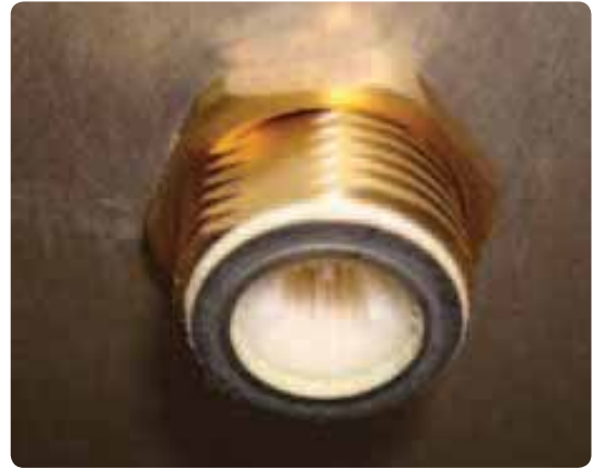
Figure 42 DHW inlet has a filter screen
