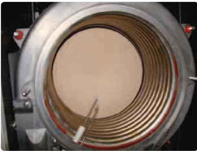
Figure 140 Inspecting and cleaning heat exchanger
