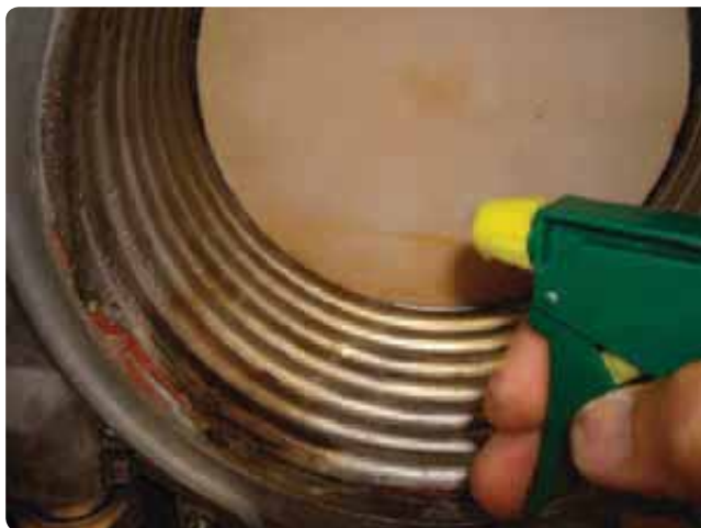
Figure 141 Cleaning the heat exchanger
