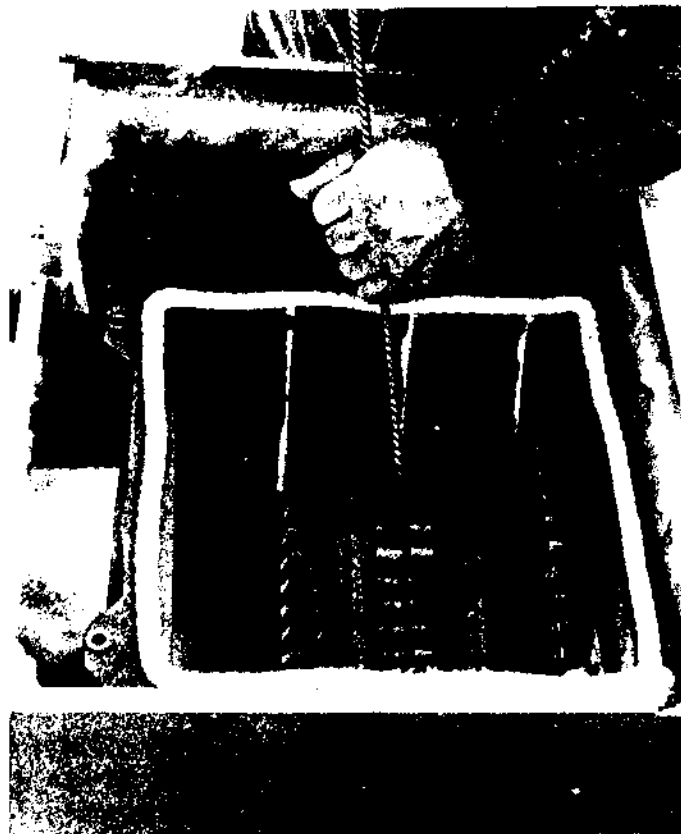
Cleaning Boiler Flueways Figure 3
