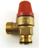
This valve is also part of the 'sealed' heating system. It is designed to operate if there is a problem with the expansion vessel or the system is over pressurised. This operates to remove pressure from the system.
