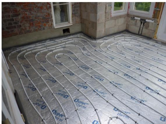
Underfloor heating is a set of plastic pipes that are often run under a solid concrete floor surface and use the floor itself to heat the room, by radiating heat upwards.
