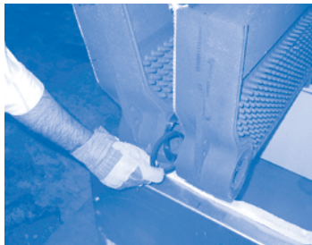
Cast iron section assembly with rope seal and gasket placement
