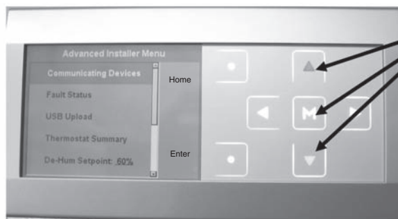
FIGURE 78 IN THE ADVANCED INSTALLER MENU SELECT COMMUNICATING DEVICES .
