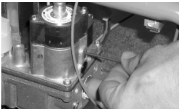
FIGURE 39 GAS VALVE PRESSURE ADJUSTMENT ( \frac{3}{32} " ALLEN WRENCH)
