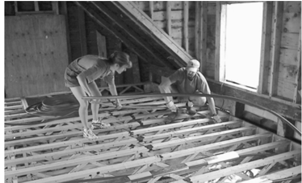
Trusses are so wide open that running 7/8" PEX through the bays becomes a very simple job.
