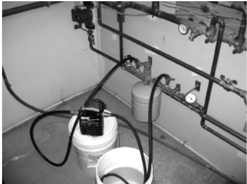
To charge a closed system with fluid, connect a ½ hp utility pump to the Expansion and Purge Kit. Immediately after starting the pump, open both the "fill" and "drain" valves, then close the "isolation" valve between them. When the system is free of air, charge the system to 15-20 psi
