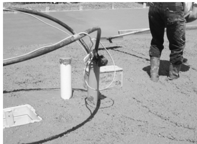
Pouring the slab around the manifold box
