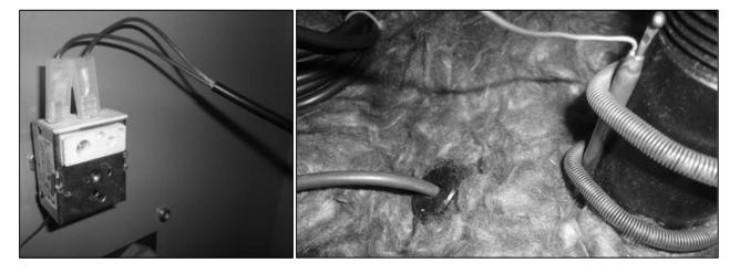
4. Draw wiring to mains and heating circuit pump through related holes on rear side of left hand panel to move them out of the boiler. Use cable clips and secure the cable and clips together on the side panel of the boiler as shown on following pictures.
