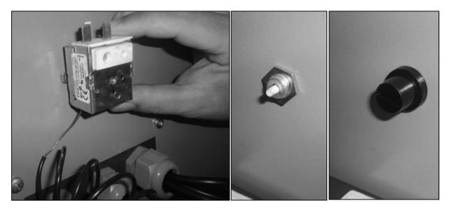
3. Attach both ends of safety thermostat wire from control panel onto terminals of safety thermostat as shown in the following picture. Attach sensing bulb of safety thermostat onto boiler hot water outlet pipe, fixing the bulb by the help of the springs supplied together with accessory pack. Attach NTC sensor of boiler thermostat (from control panel) into the pocket phial on top of the boiler body in front of hot water outlet pipe.
