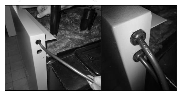
5. Take wiring from the control panel to the fan whose end is connected to 4 plug female socket. Attach this socket to the right hand side panel of the boiler, as seen in the following picture.
