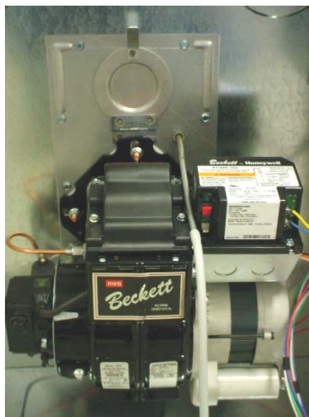
Figure 6: Checking Over-Fire Draft.
