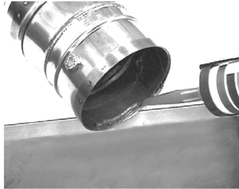
Applying bead of silicone to the female portion of the appliance / vent adaptor.
