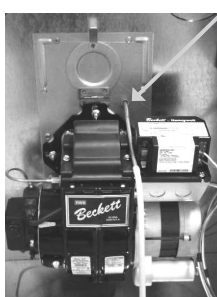
Over-fire draft access port.
