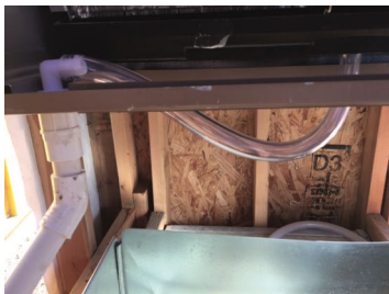
Figure 21: Condensate-tube installed
