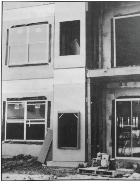
Figure 9: Wall sleeve installed from outside angle 1
