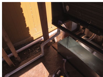
Figure 22: Condensate-tube installed
