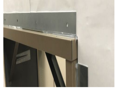
Figure 17 - Caulk seal outside joints of wall sleeve before inserting into wall opening (Underside view of wall sleeve bottom).
