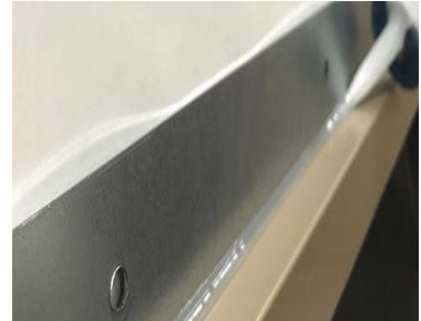
Figure 18 - Caulk seal outside joints of wall sleeve before inserting into wall opening.
