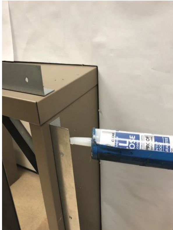
Figure 16 - For additional protection against air infiltration during periods of very high winds, fill the clearance space between unit and wall sleeve all around with sealant.
