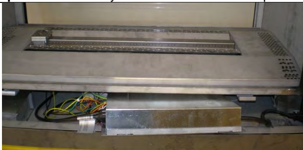
Remove Glass Doors from both sides of fireplace. Remove UHS Box from bottom of fireplace.
