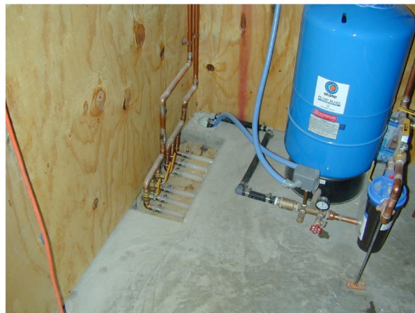
Slab manifold fully installed with box broken apart
