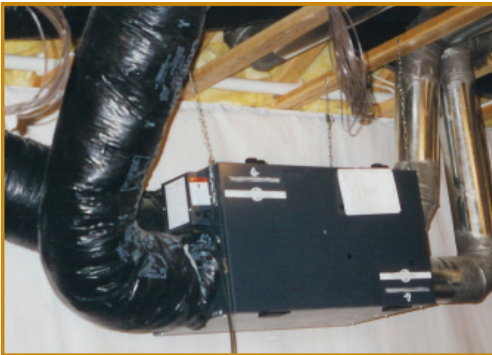
Figure 13-A. Typical installation of a heat exchanger. (Photo courtesy of Shirley Neimayer, University of Nebraska - Lincoln).
