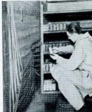
Heating cable installed in moist-room used in testing samples of concrete
