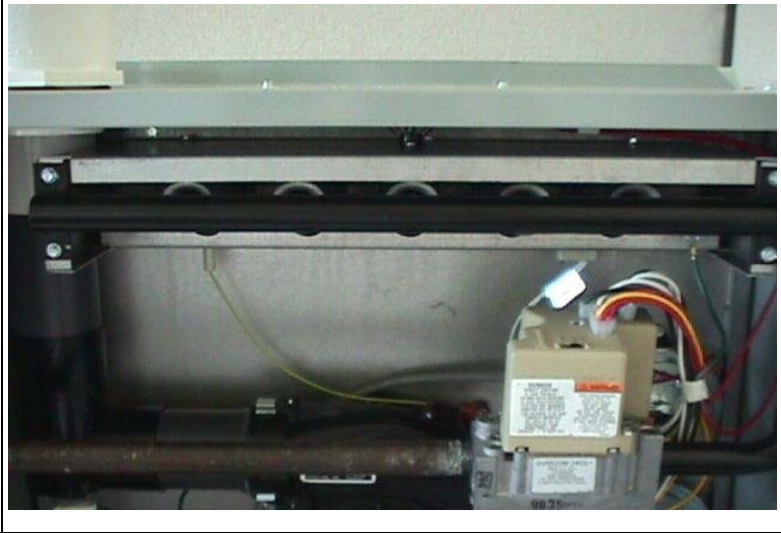
Figure 30: Inshot Burner Assembly
