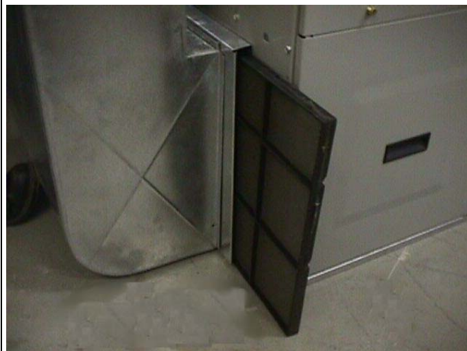
Figure 22: Air filter Maintenance.
