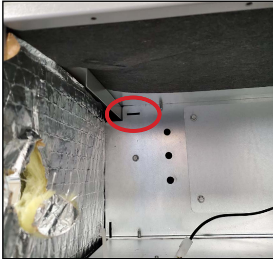
Figure 12. Notch for Control Panel Relocation
