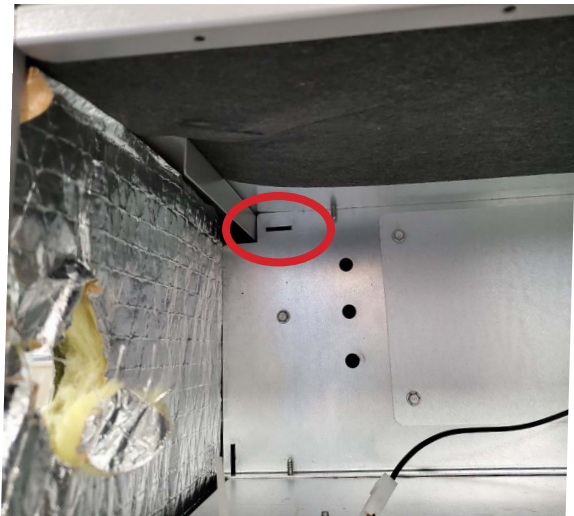
Figure 12. Notch for Control Panel Relocation
