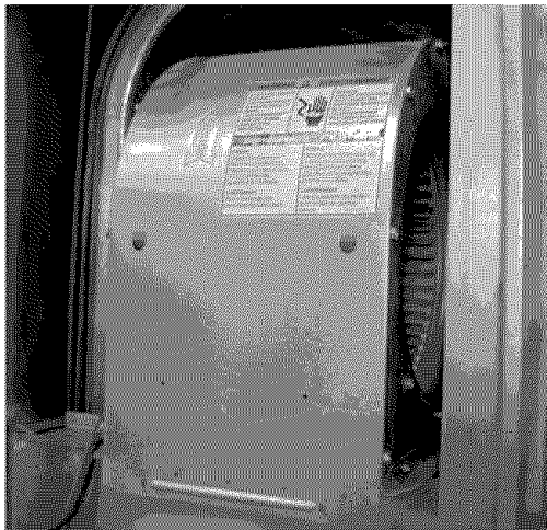
FIGURE 45: Install and secure blower on shelf. Plug blower motor into control box.
