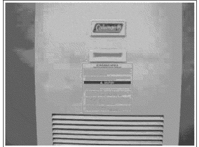
FIGURE 50: Install Consumer Notice on top front furnace door and instruct the consumer on how to properly maintain their furnace.
