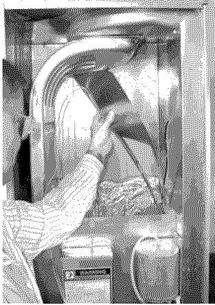
FIGURE 37: Bow back plate of auxiliary limit switch assembly to insert on right-hand side of blower compartment.
