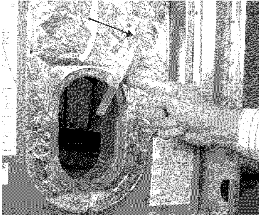
FIGURE 25: Reposition air vane to original position. Reinstall bottom screw and tighten top screw.
