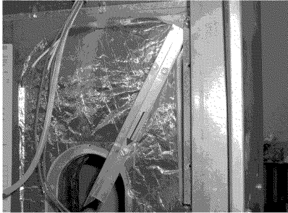
FIGURE 13: Remove bottom screw from air vane, loosen top screw and rotate air vane counterclockwise. Use caution when rotating air vane so that foil faced insulation is not damaged.
