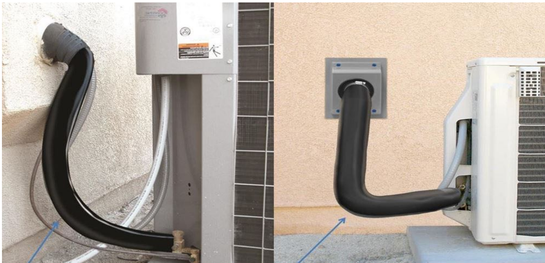
Figure 4-1: Refrigerant Line Insulation
