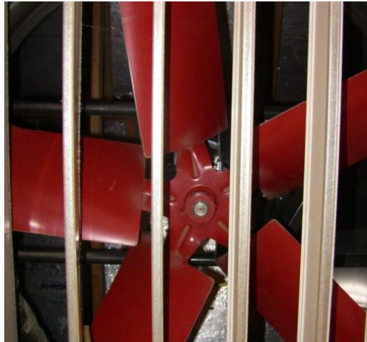
Figure 4-39: Open Barometric Damper With Fan Above
