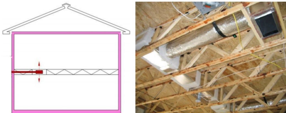
Figure 4-13: Open Web Floor Truss Example
