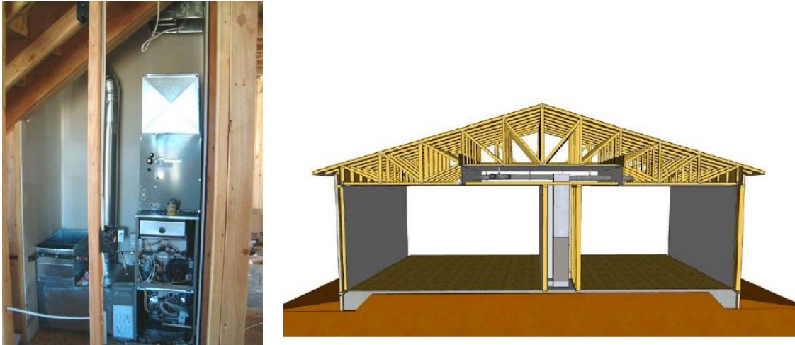
Figure 4-14: Mechanical Closet Placement Example
