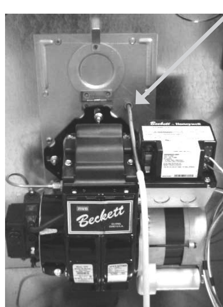
Over-fire draft access port.
