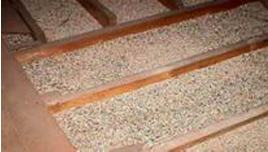
Vermiculite insulation between attic joists
