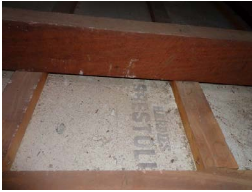
Photo 1: Rear side of LDB ceiling sheet showing trade name.
