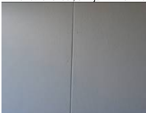
Photos 9 and 10: Examples where fasteners are fixed into the LDB sheeting and the edges are bevelled or slanted.
