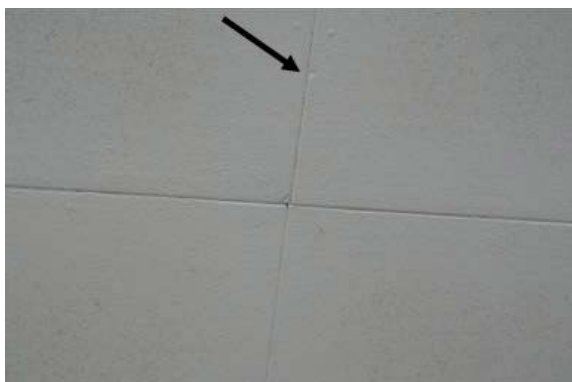
Photo 7: Recessed fastener heads in LDB.
