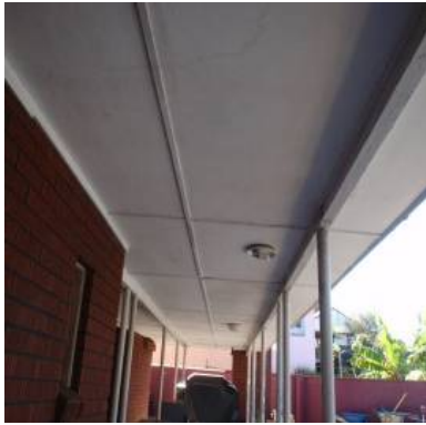
Photo 11: Asbestos cement sheets joined with timber cover strips.
