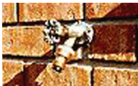
Figure 9.17. Hose Bib With Vacuum Breaker
