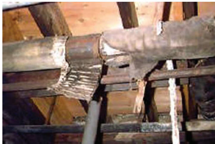
Figure 12.6. Heating Ducts Covered With Asbestos Insulation
