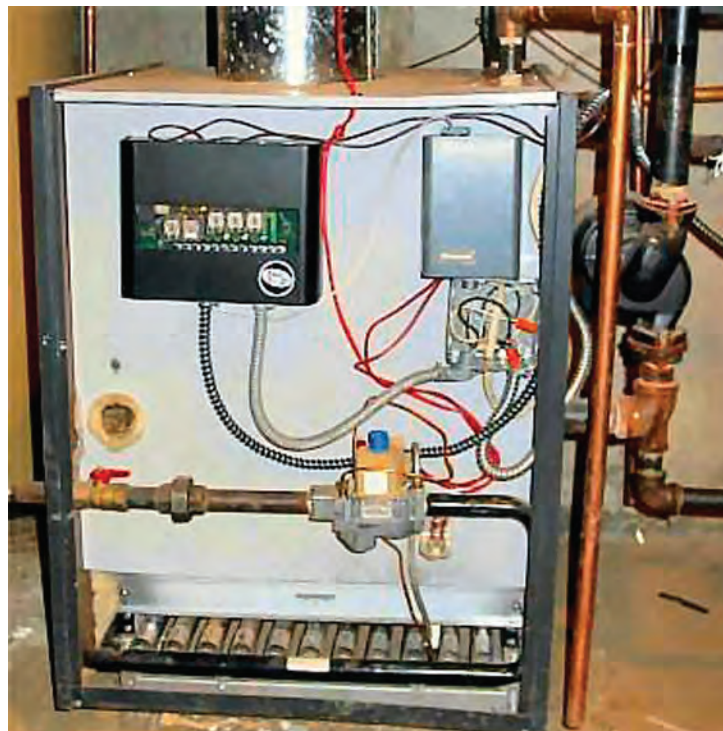
Figure 12.9. Gas-fired Boiler
