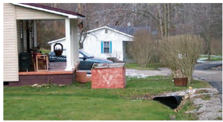
Figure 8.7. Typical Dug Well
