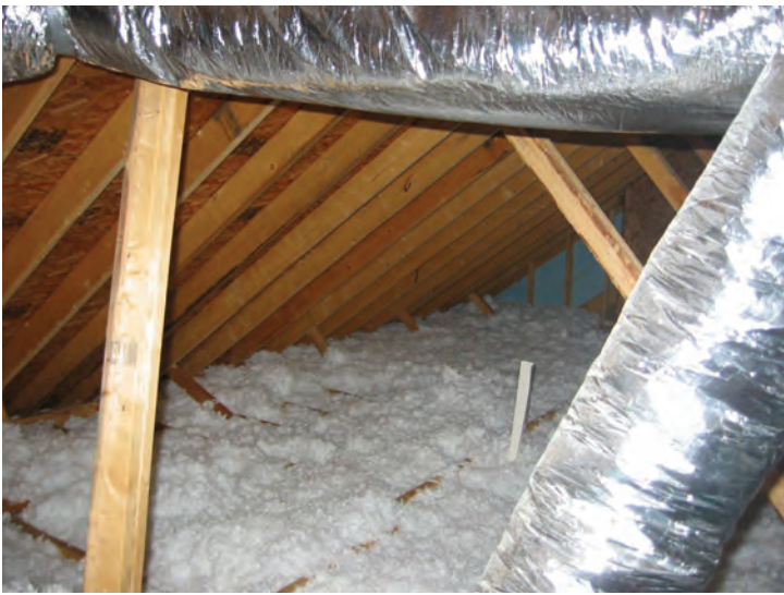
Figure 7.2. Blown Attic Insulation
