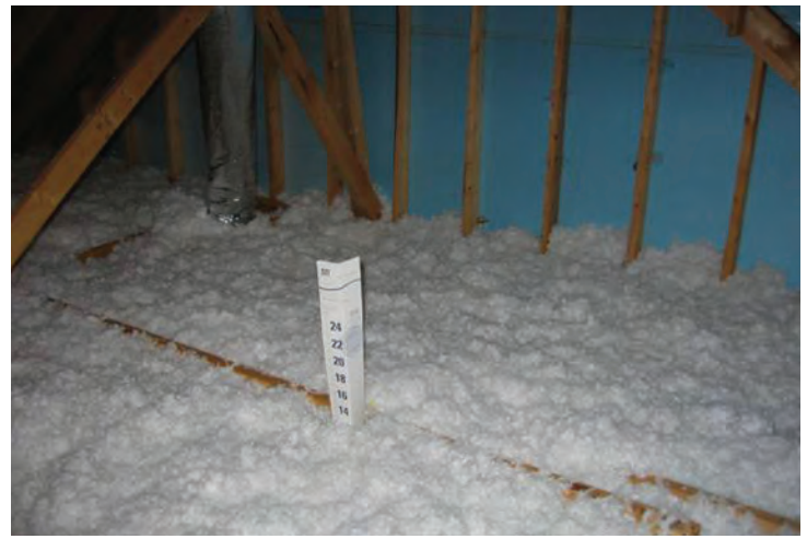
Figure 7.3. Depth of Attic Insulation
