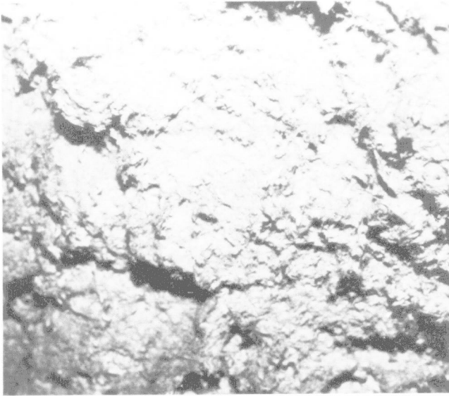
Friable, fluffy sprayed-on material
