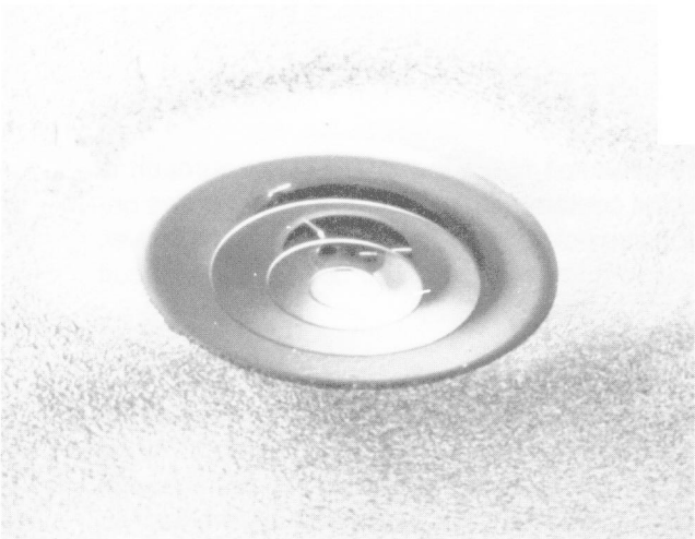
Airstream erosion from a heating vent
