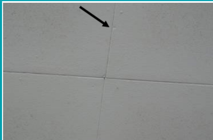
Figure 6 Recessed fastener heads in LDB
