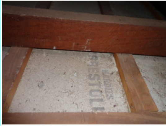
Figure 1 Rear side of LDB ceiling sheet showing trade name
