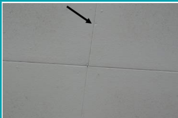
Figure 6 Recessed fastener heads in LDB
