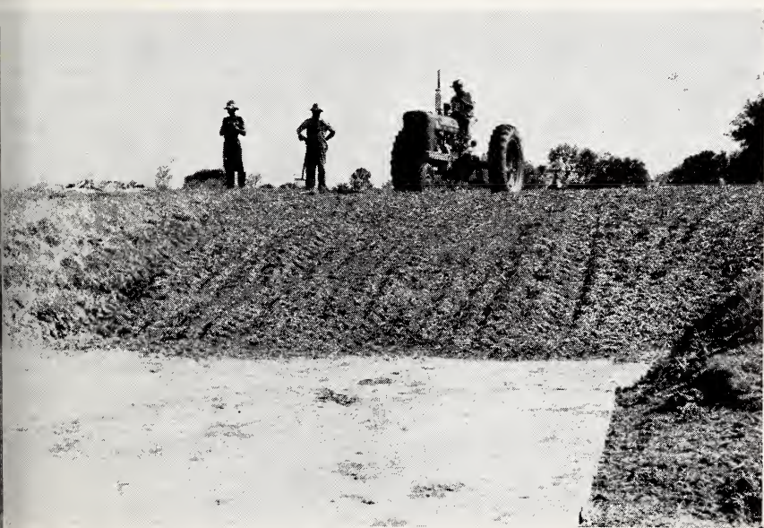
Fig. 16.—Packing an earth bank bunker silo with a farm tractor.
