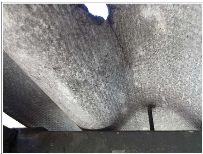
Figure 23: Fiber Cement Plate Fracture. Despite not being a friable material, the deterioration of this material implies the release of fibers and its consequent danger for people who are in the environment, so it is necessary to remove asbestos (author's Photograph)
