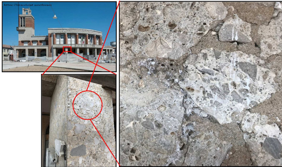
Figure 5. Concrete infilling mortar sample CO3. The Ex casa del Fascio building has been affected by damages caused by the earthquakes in May 2012, but before these events it was been subjected to restore operations not always made following the correct procedures for historical building.
