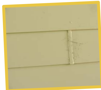
Hardi plank wall sheeting
