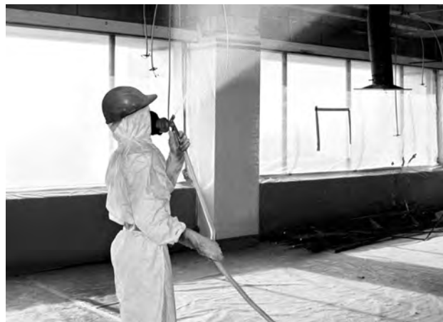
Figure 34-4: Spraying ACM with Amended Water Before Wet Removal
