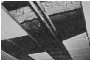
Suspended Ceiling Concealing Fireproofing
