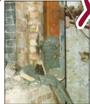
Sprayed asbestos (limpet)
