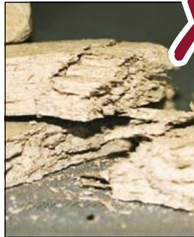
Broken asbestos insulating board
